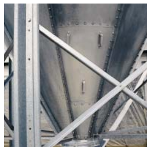
▲ The E-Z Kleenout panel can be easily adapted to existing feed bins.
